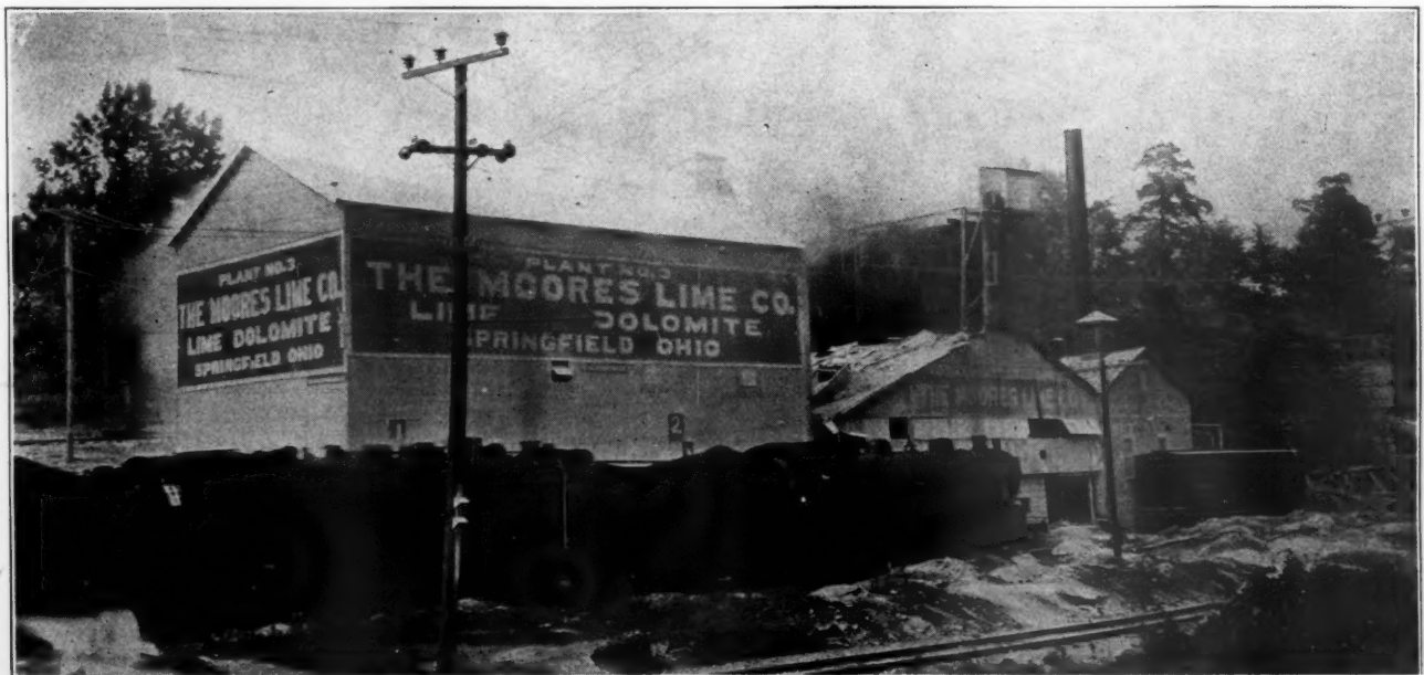
Hydrating and Lime Plant
